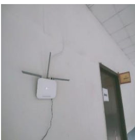
Thatta New Internet Router Install For Strong Internet Connectivity
