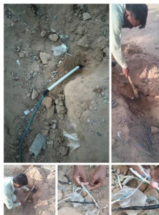
Camera Maintenance & Cleaning CCTV camera underground wire repairing.
